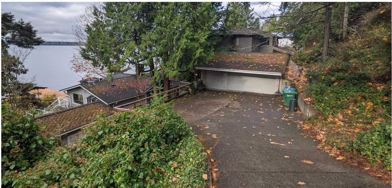
Plate 4. General conditions of the driveway apron and existing garage, looking north.
