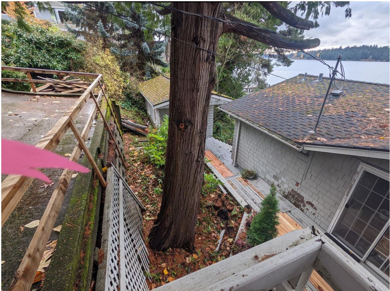
Plate 3. General conditions between the existing residence and driveway apron, looking south.
